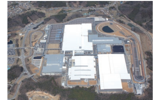
Saitama Factory Automobile Plant
