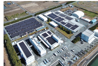
Hosoe Outboard Engine Plant (1.7 MW)
