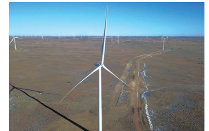
Boiling Springs Wind Farm (120 MW)
